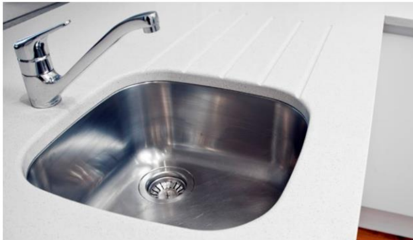
Undermount Sink Installation
